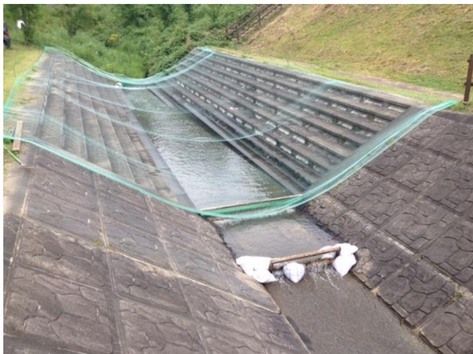
Figure 1-10 Picture of installation case of zeolite sheet. The decontamination was carried out by Toppan Printing Co., Ltd.
