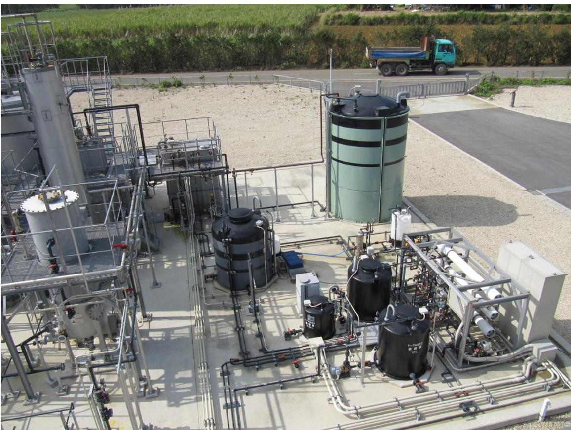
**Fig. 6-3** Photo of full-scale physicochemical treatment processes
