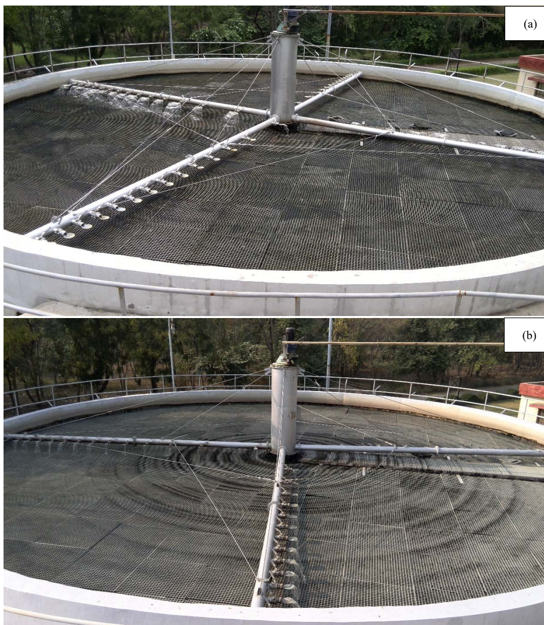
Fig. 7-1 Picture of sprinkling wastewater of the DHS reactor ((a) 5,000 \text{ m}^3 \text{ day}^{-1} (2 arms), (b) 3,000 \text{ m}^3 \text{ day}^{-1} (4 arms))
