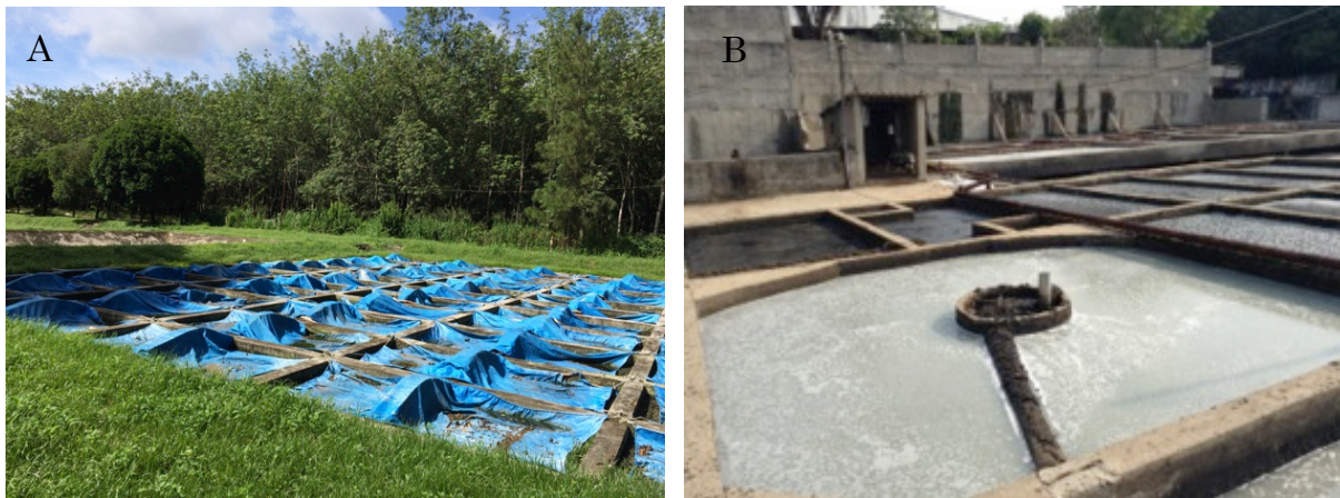
Figure 2.5 anaerobic biological pond in (a) Rubber Research Institute of Vietnam (b) Mia Thao Rubber sheet processing factory.
