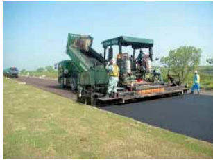
Figure 2. Spreading the asphalt mixture
