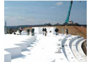
Photo 3. EPS method (Source: Nagaoka National Highway Office)
