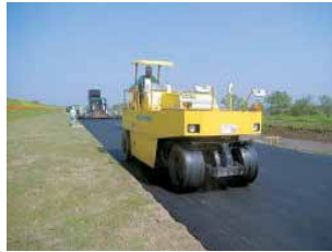
Figure 3. Compacting the asphalt mixture
