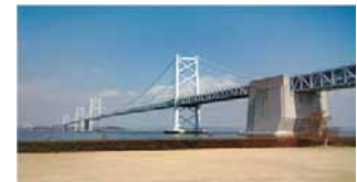
Photo 6. Great Seto Bridge (1,723 m in length, built in 1988)
