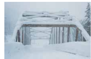
Photo 3. Arch bridge with snow accumulation
