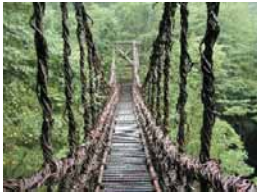
Photo 3. Kazura Bridge in Tokushima prefecture
