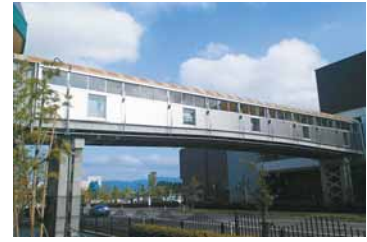
Connecting bridge at Riverside Senshu shopping center
