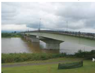
Photo 1. Girder bridge in Nagaoka
