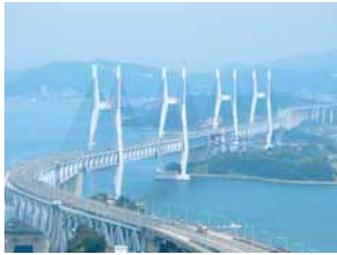
Photo 4. Cable-stayed bridge connecting an island in the Seto Inland Sea
