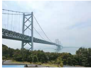
Photo 5: Suspension bridge connecting an island in the Seto Inland Sea
