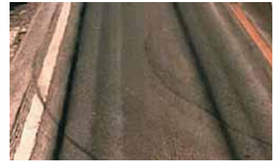
Figure 1. Serious rutting
