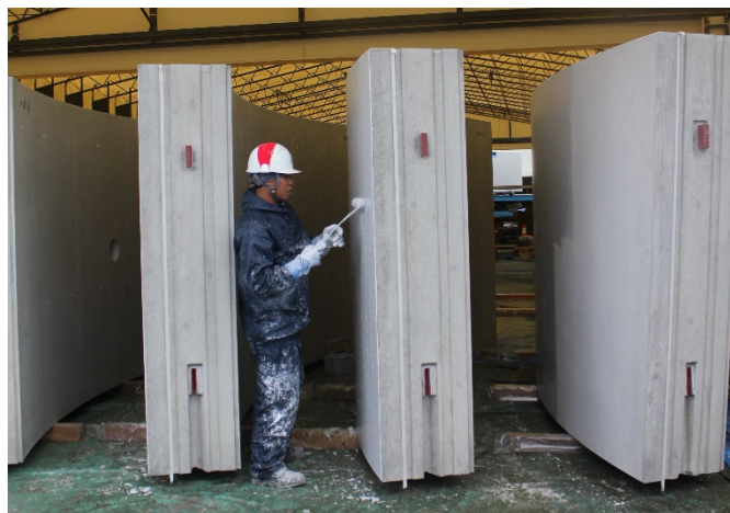
Figure 2.1. Coating outer surface of segments.
