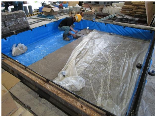
(c)粘性土路盤の敷設
